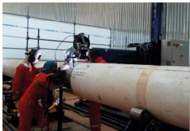
Fig.2: Welding set on a boom end
