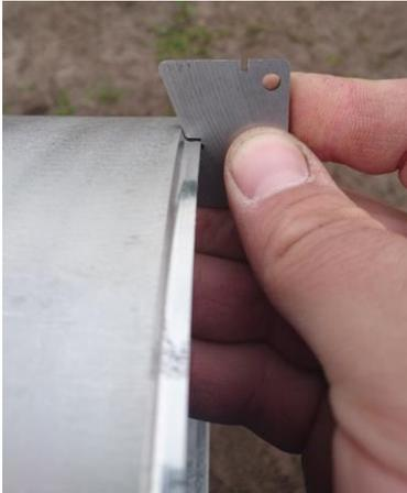
*Fig. 8: Correct pipe end preparation is carried out on site before the welding operation and checked by means of a template*
