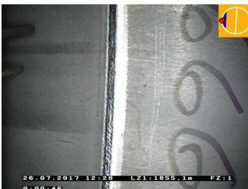
*Fig. 9: Capture from a video of the blank metallic surface at the inside of the joint (welding shown in Fig. 6)*
