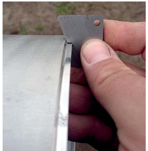
Figure 7. Correct pipe end preparation is carried out on site before the welding operation and checked by means of a template
