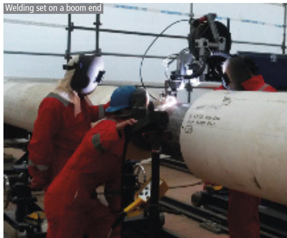
Welding set on a boom end
